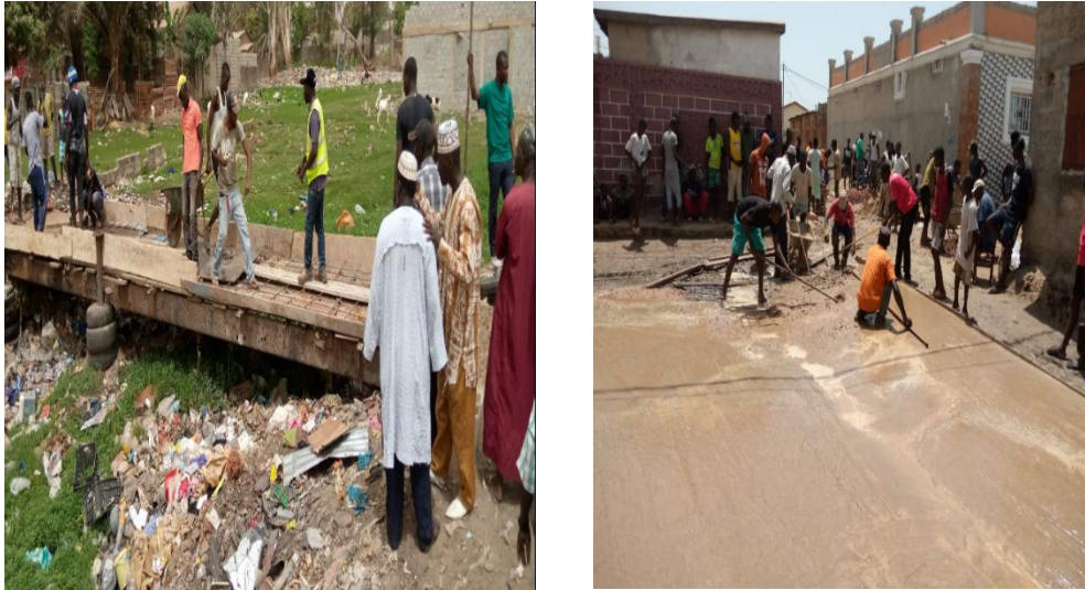
Figure 20. Members of the Community Participating in the Construction of a Foot-Bridge
