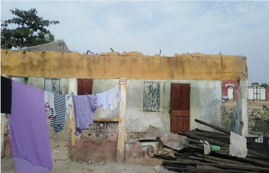
Figure 7. A House Destroyed in Ebo Town during the 2022 Windstorm
